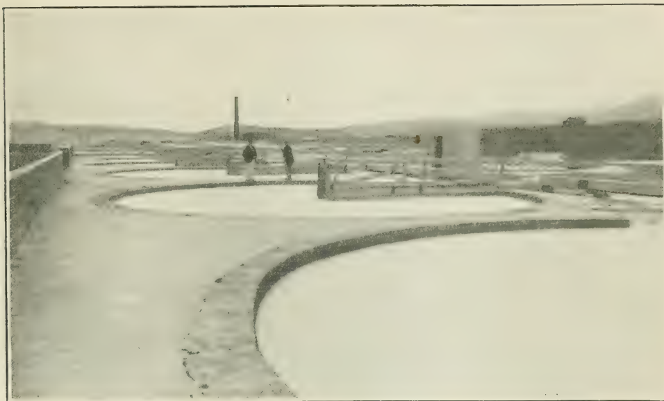
FIG. 8. ROW OF SETTLING PITS. (Photo, English China Clays, Ltd., St. Austell. )
